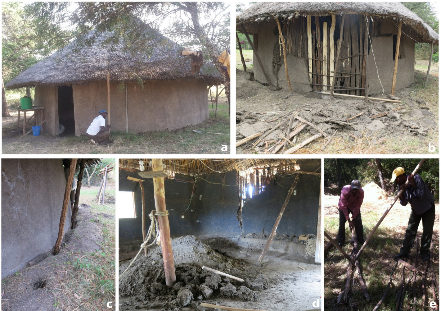
Figure 6: a) The camp's main tukul (used as a dining room); b) the tukul during the initial stages of restoration, showing the temporary roof support, the detached daub and the wooden framework of the wall; c) detail of the temporary roof supports, showing the holes in which the poles were sunk and the ring of earth that accumulated around the base of the wall; d) the interior of the tukul, showing how fragments of the old daub accumulated on the floor; e) splitting poles for the new wall.
